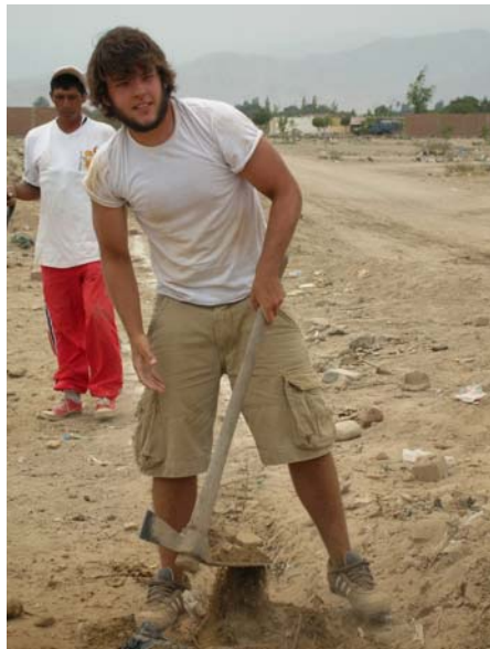
Corvallis' own Jesse Bontrager helping at Peruvian construction site.
