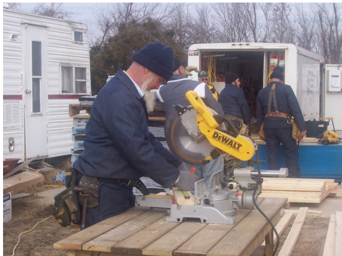
Transforming a Trailer: Many hands make light work.
